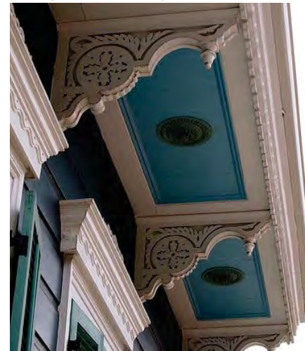
Overhang/Bracket detail at porch
