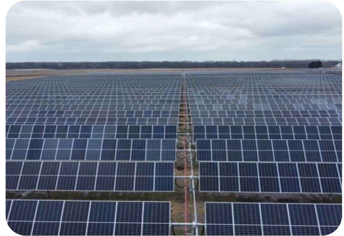
Apex's Coldwater Solar PV generation facility in Branch Co., Michigan.
