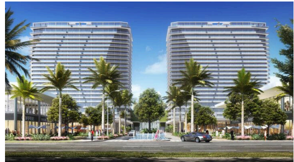
Oasis East and West Towers in Hallandale Beach, Florida
