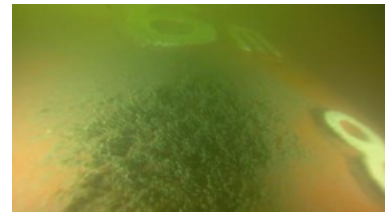
Coating adhesion failure
